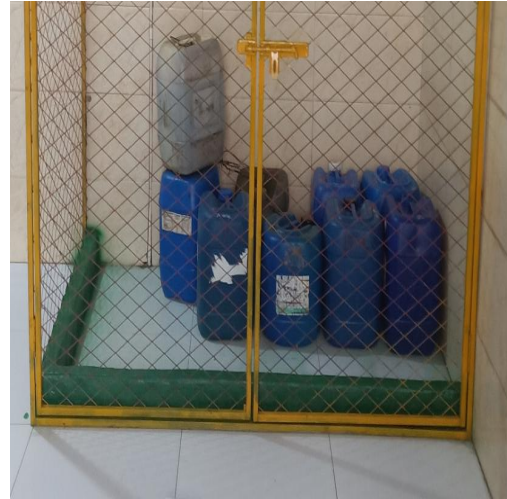
危废暂存区围堤
