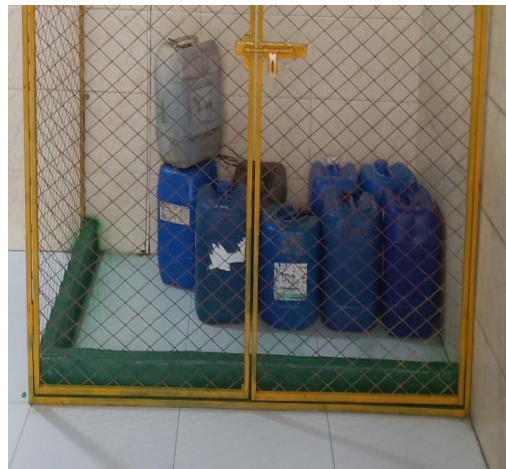
危废暂存区围堤
